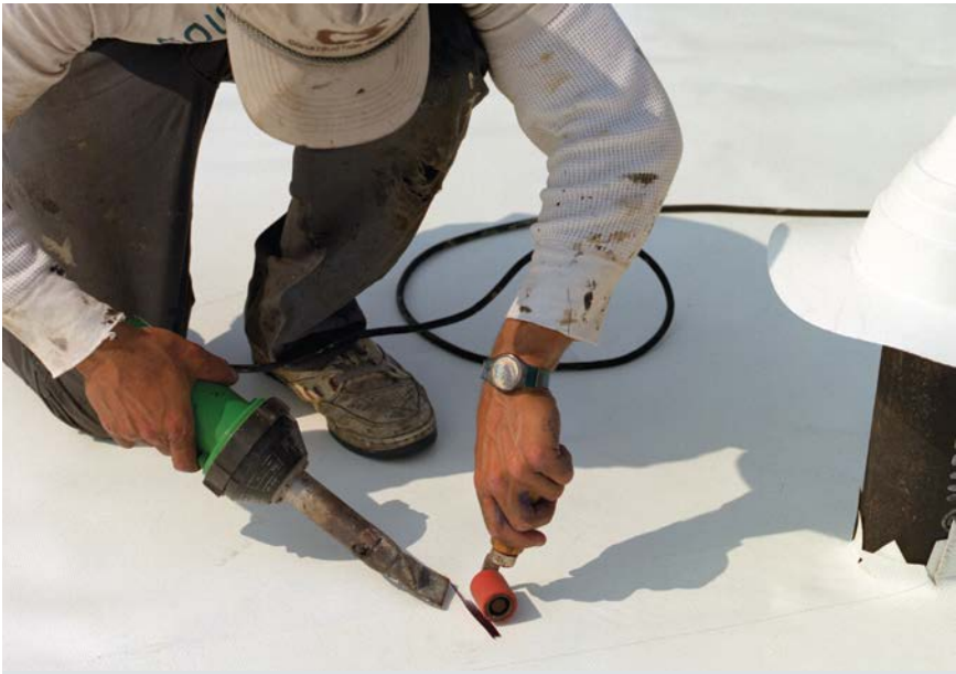
Cool roofs can be made of either white or darker colored materials. While white roofs are usually cooler, both will reflect near-infrared sunlight and save energy and money.
