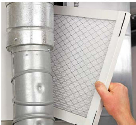
Clean or replace furnace filters once a month or as needed.
